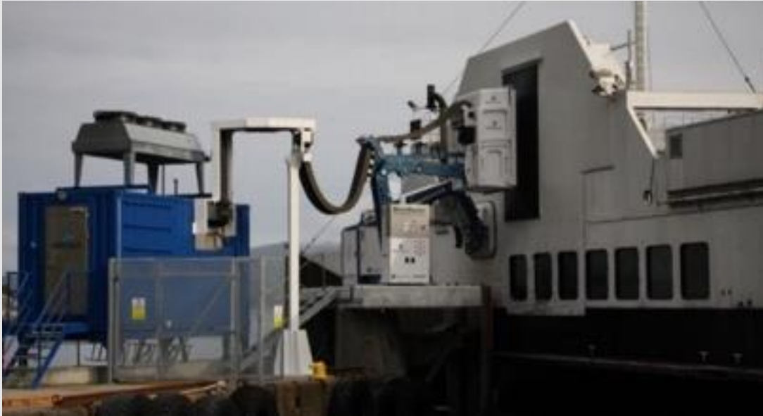
Inductive and plug charging solutions developed and tested onboard Folgefonn
